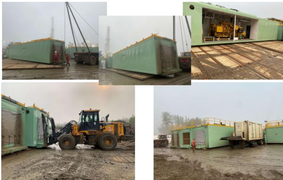
Figure 12: Natural Gas Engine Buildings Unloading at Project Rig #1
